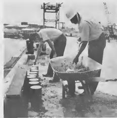
CORE SAMPLES were taken throughout the big pour. The hopper rider and vibrator man had unusual tasks.
